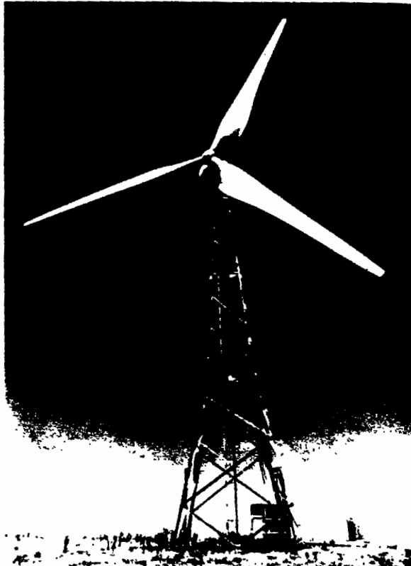
Three one-ton turbine blades sweep through a 108' diameter circle.
