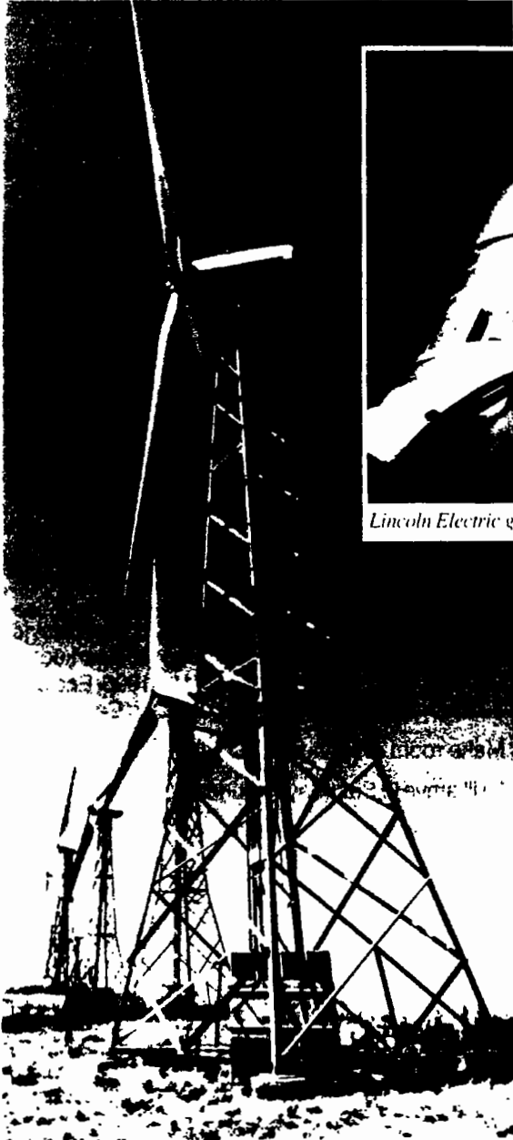
Turbine towers range in height from 80' to 120'
