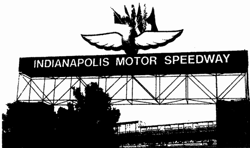
Newly refurbished Speedway entrance.
