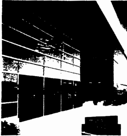
The current Lincoln Electric Company headquarters building in Euclid, Ohio.
